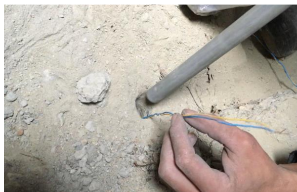
Fig. 6. Loading of the charge in the blast-hole
