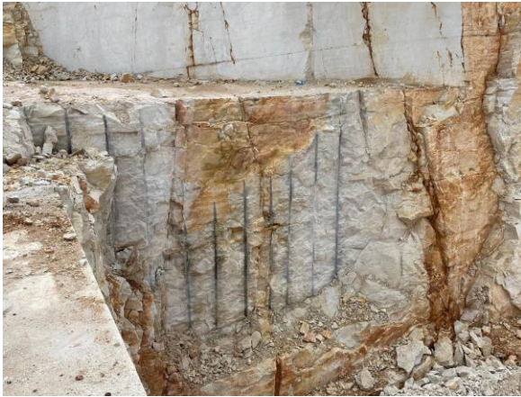
Fig.7. Effect of smooth blasting on the limestone wall after excavation
