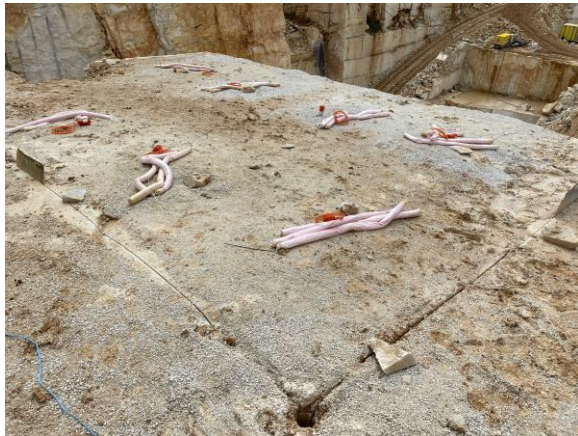
Fig.11. Pre-cutted along the perimeter block of overburden, repaired for loading with explosives.
