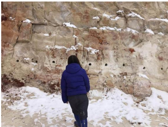
Fig.8. Horizontal drill holes for pre-split blasting
