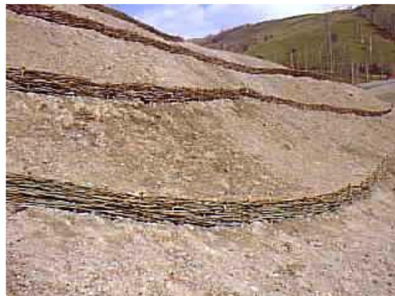
Fig. 1. Work to prevent soil erosion and to drain the dripping waters
