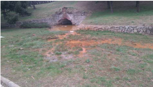
Fig. 4. Water surface inflow through the exit of mining gallery MG-1 in the region of Pernik neighborhood Dimova mahala
