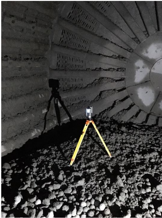
Fig. 2. The laser scanner during a measurement
