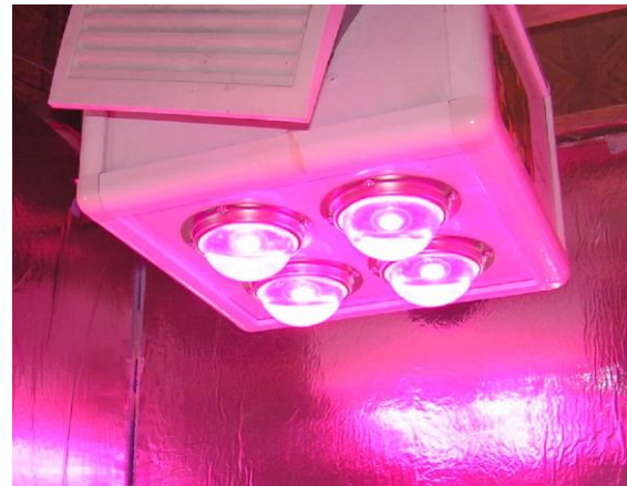
Fig. 11. Cabin No 6 - Specialised luminaire designed for photosynthesis
