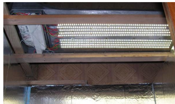
Fig. 12. Cabin No 7 - Illumination light emitting neutral white light - 4337 K (control)
