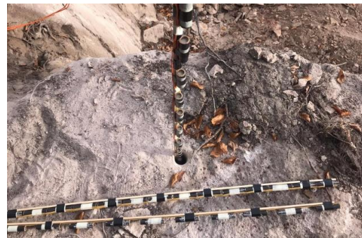
Fig. 8. Field test with decoupled chain-charges for smooth splitting at stone quarry
