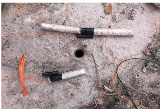
Fig. 10. Ready for loading charges of propellant-based non-detonating compositions
