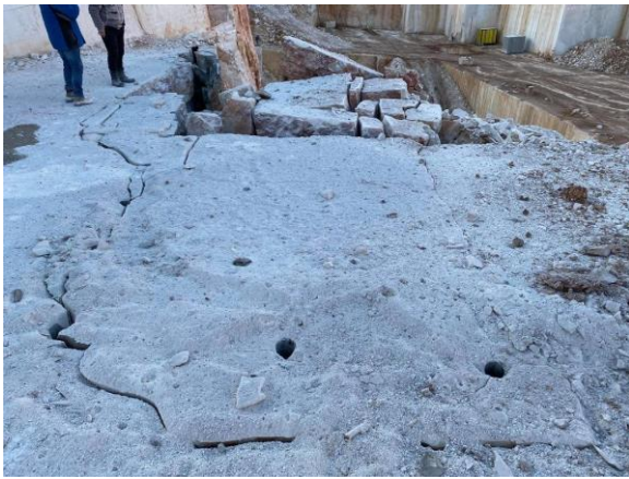
Fig.6. Pre-splitting crack and displacement of the low quality limestone after split-blasting
