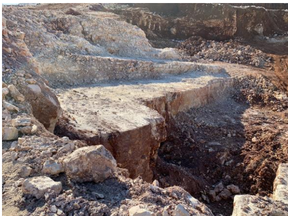
Fig.2. Bench blasting for removal of waste rock in dimension stone quarry
