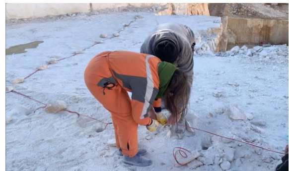
Fig.4. Pre-split blasting preparation
