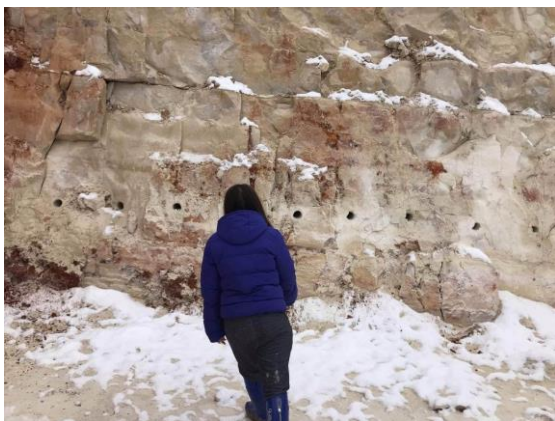
Fig.8. Horizontal drill holes for pre-split blasting
