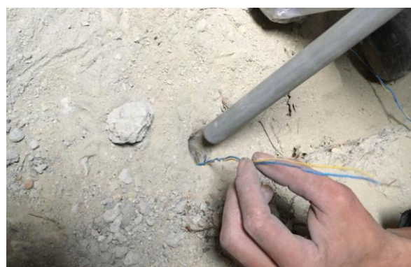
Fig. 6. Loading of the charge in the blast-hole
