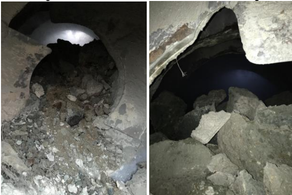
Fig. 7. Swelled concrete inside the mixer interior after blasting
