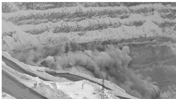
Fig. 1. Blasting works in a real open pit
