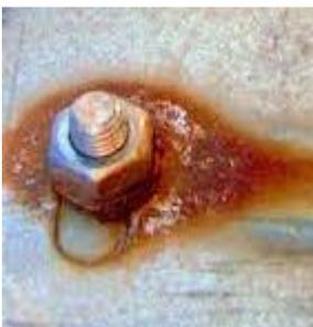
Fig. 18. Galvanic corrosion
