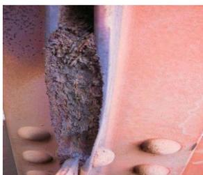
Fig. 17. Compacted rust
