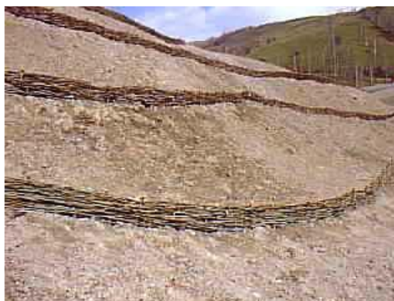
Fig. 1. Work to prevent soil erosion and to drain the dripping waters
