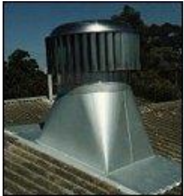
Figure 4. Outside view of turbine fan
