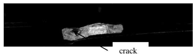
Figure 6. Crack formed on the specimen surface.
