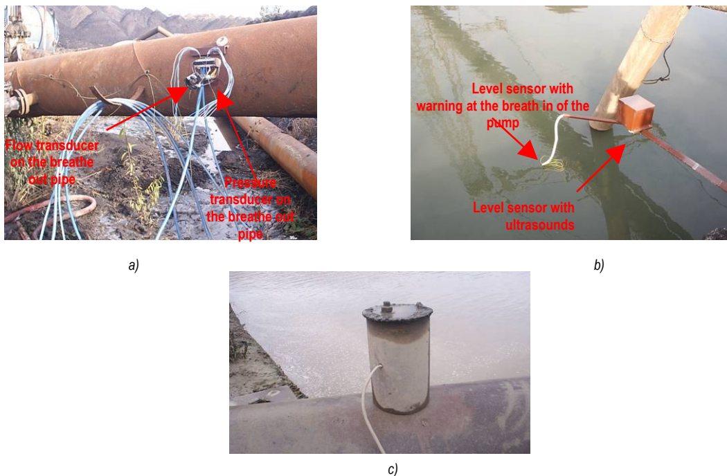
Figure 2. Mounting of the sensors: a) Mounting the volume and pressure transducer on the breathe out pipe; b) Mounting the level sensor with ultrasounds and which also warns at the pump's breathe in; c) Mounting the depressurization sensor.
