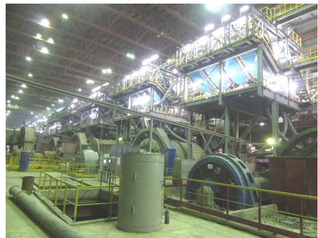
Fig. 1. The crushing unit at ANOF-3 after revamp
