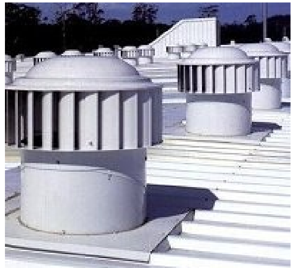
Figure 6. Actual building with roof fans
