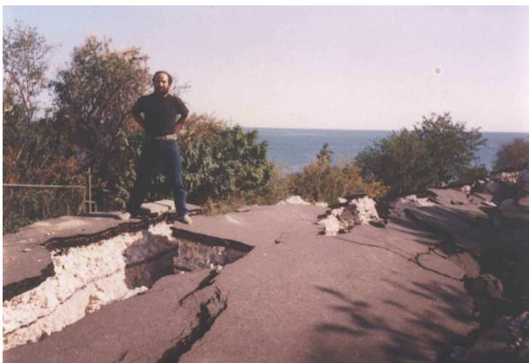
Fig. 3. Landslide in the surrounding of Varna City that destroyed the highway between the City and the resort Golden Sands
