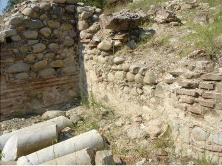
**Fig. 1. River boulders from granite and porphyry granite – from the walls of the Basilica**
